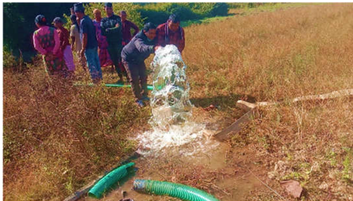
Lift Irrigation Installation in Dang
